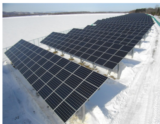
(8) Ichigo Yubetsu Baro ECO Power Plant
