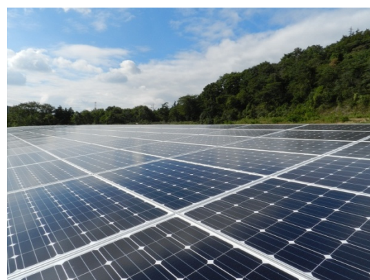
(2) Ichigo Kiryu Okuzawa ECO Power Plant
