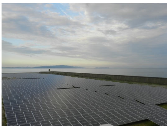
(1) Ichigo Tokushima Higashi-Okinosu ECO Power Plant
