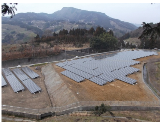
(7) Ichigo Iyo Nakayamacho Izubuchi ECO Power Plant
