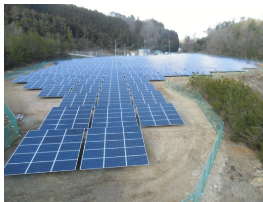
(6) Ichigo Fuchu Jogecho Yano ECO Power Plant
