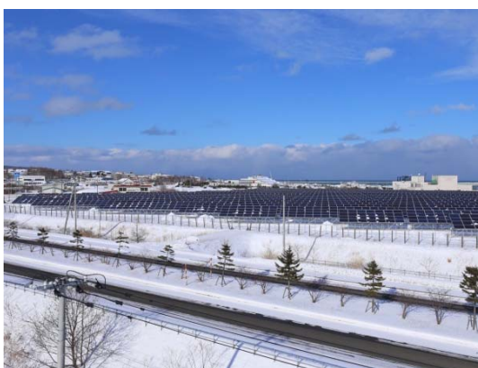
(3) Ichigo Motomombetsu ECO Power Plant
