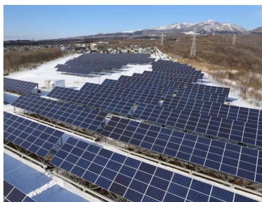
(4) Ichigo Muroran Hatchodaira ECO Power Plant
