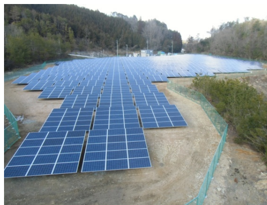
(6) Ichigo Fuchu Jogecho Yano ECO Power Plant
