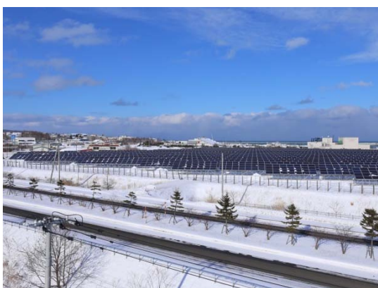
(3) Ichigo Motomombetsu ECO Power Plant
