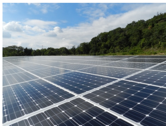
(2) Ichigo Kiryu Okuzawa ECO Power Plant
