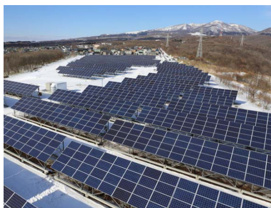
(4) Ichigo Muroran Hatchodaira ECO Power Plant
