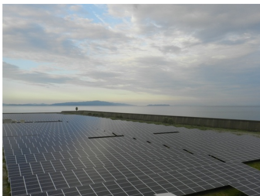
(1) Ichigo Tokushima Higashi-Okinosu ECO Power Plant
