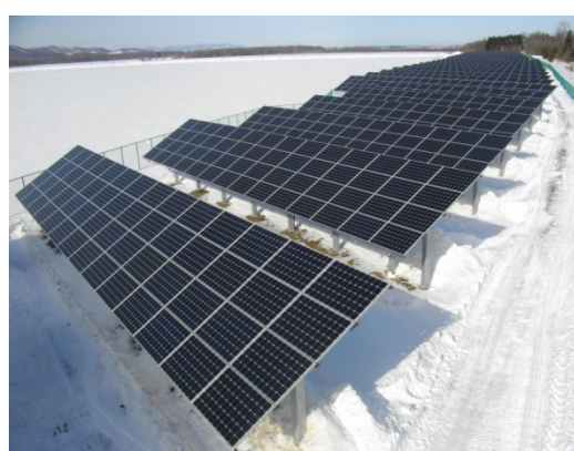
(8) Ichigo Yubetsu Baro ECO Power Plant
