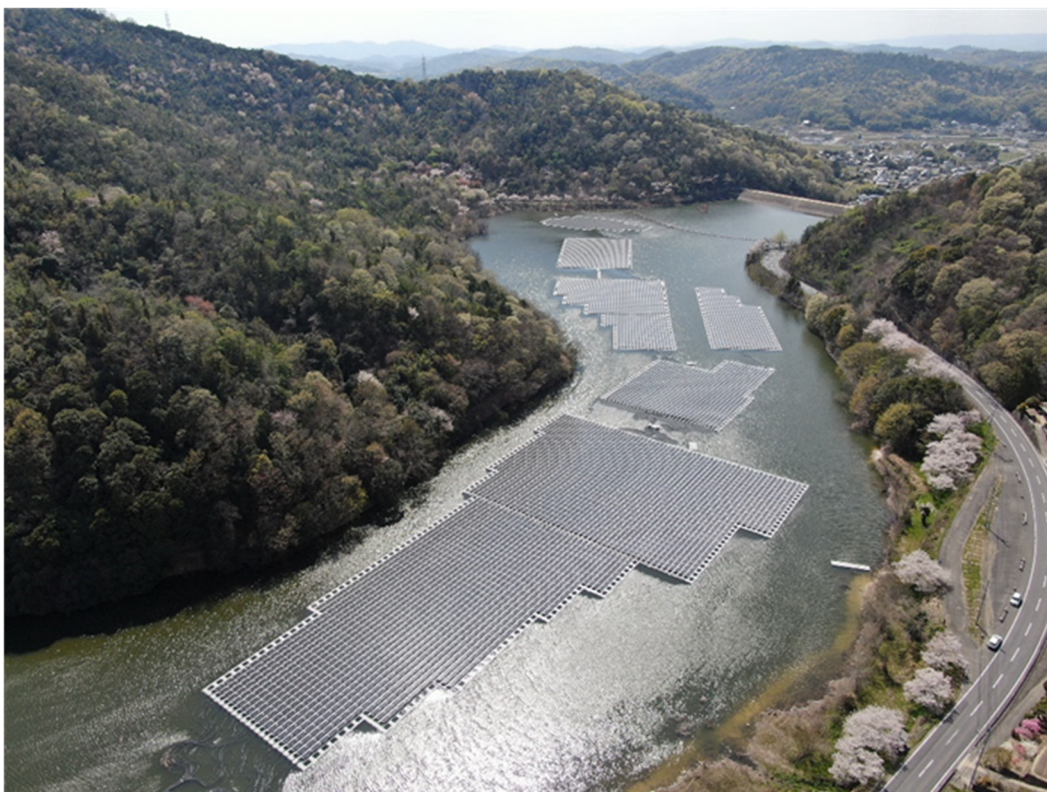
Ichigo Kasaoka Osakaike ECO Power Plant
