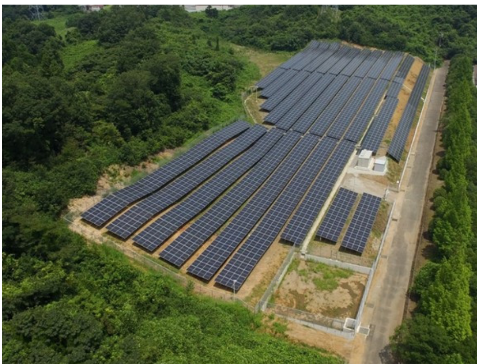
Ichigo Minokamo Hachiyacho Kamihachiya ECO Power Plant
