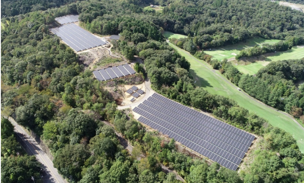
Ichigo Seto Jokojicho ECO Power Plant
