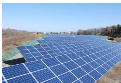
Ichigo Abira Toasa ECO Power Plant
