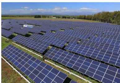
Ichigo Nakatshibetsu Midorigaoka ECO Power Plant
