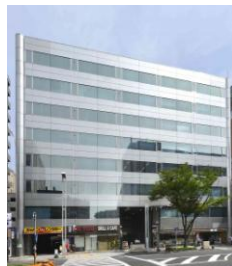
Ichigo Nagoya Building
