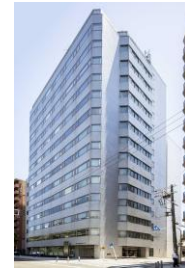
Ichigo Nishi Honmachi Building
