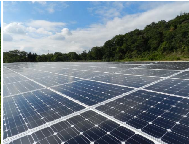
Ichigo Kiryu Okuzawa ECO Power Plant (1.33MW)
