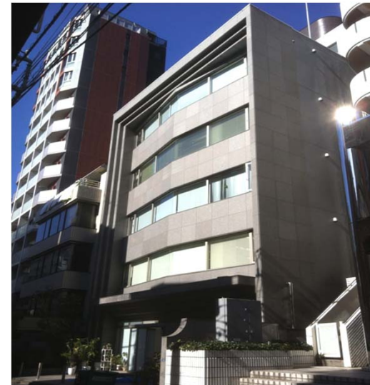
Five-story office building with basement acquired in March 2015 Conducted 1-year value-add and completed sale to investor in October 2016
