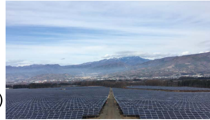
Ichigo Showamura Ogose ECO Power Plant
