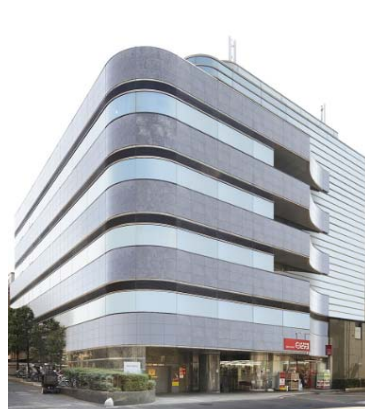
Ichigo Hongo Building
