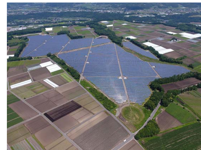
Ichigo Showamura Ogose ECO Power Plant
