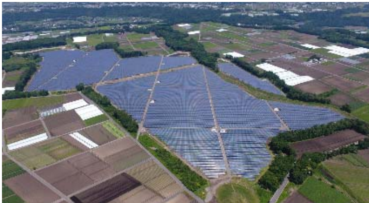
Ichigo Showamura, Tokyo's Largest Solar Power Plant
