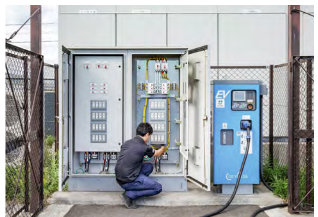
Ichigo engineer Suwabe checking the emergency charging station at the Ichigo Kasaoka Takumicho ECO Power Plant.
